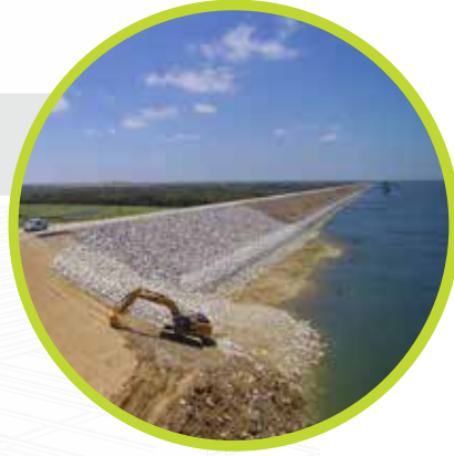
River Bank Protection
