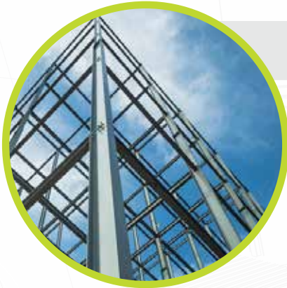
Specialized RCC/ Steel Structure
